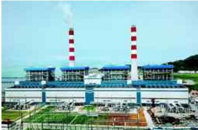
Yuhuan, China, coal-fired plant with super-critical steam turbines 4 x 1000 MWe, 45% efficiency. NB: supercritical steam is much more efficient at driving the giant turbines that spin the plant's generators.
