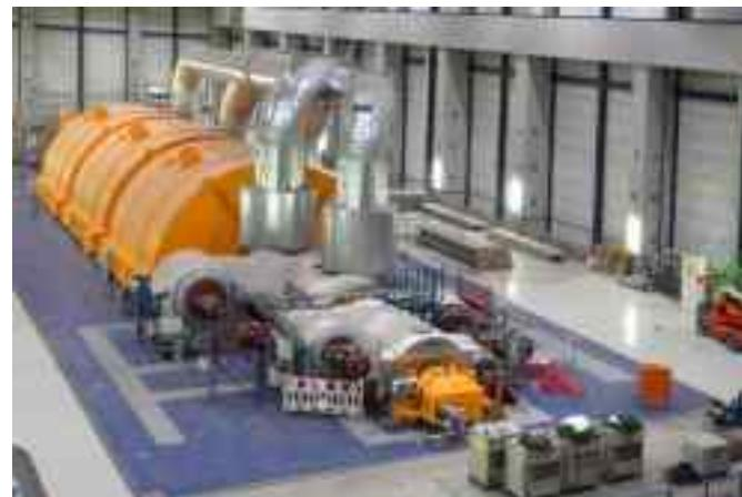
Germany, Ultra-SuperCritical steam (USC) power plants. This technology is operational at a new coal-fired power plant. Operated by German utility EnBW, the plant achieves 47.5% net thermal efficiency while producing 912MW of electricity, making it one of the world's most efficient hard coal-fired steam power plants.
